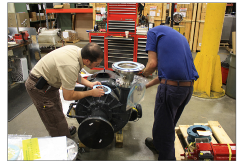
The Hope Group engineers and technicians recently built and installed a renewable energy system for the Keene, NH community at its Water Treatment plant.
