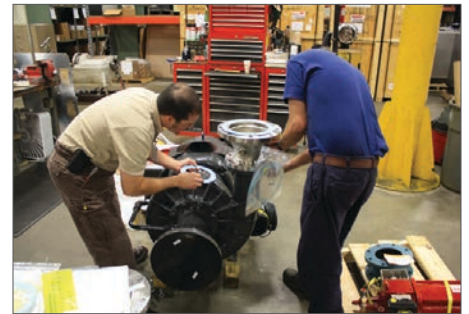
Sorensen Systems engineers and technicians recently built and installed a renewable energy system for the Keene, NH community at its Water Treatment plant.
