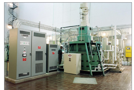
The Hope Group built two new digital excitation control systems as part of refurbishment.
