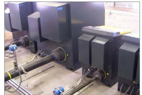
*The ambient air, gravity-fed system needed a boost from the low-pressure blowers as demand for propane gas increased from residential and commercial expansion.*
