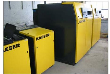
*The four low pressure blowers installed at NH Gas in Keene NH were designed to cover a wide cfm range and to serve as internal back-up during routine maintenance.*
