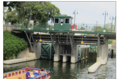
Sorensen Systems and Steel Fab worked together to design, build and install two sets of miter gates and a crest gate at the San Antonio River Walk.
